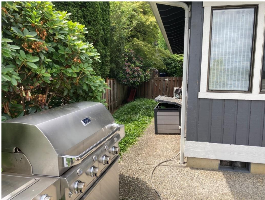
Plate 3: View of proposed south side hallway area, looking west from southeast corner of existing house.
