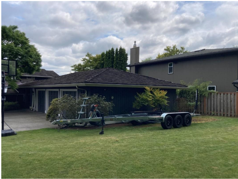
Plate 1: View of existing detached garage, looking southeast.
